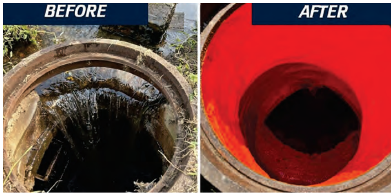
Example of a relined manhole barrel to reduce infiltration.
